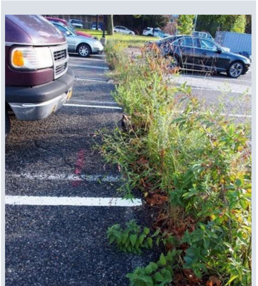
Parking lot with permeable pavement and grade level rain garden medians. Photo credit: Columbia University 13
